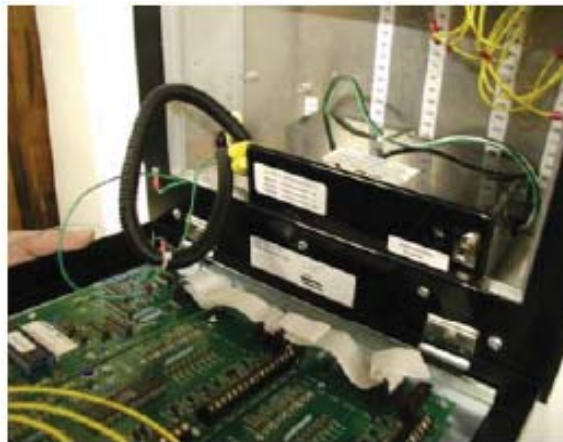
Inside view of a nearly completed conversion
